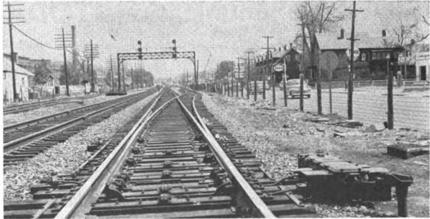
Track 3 was removed from old SS-22 to Riverside
