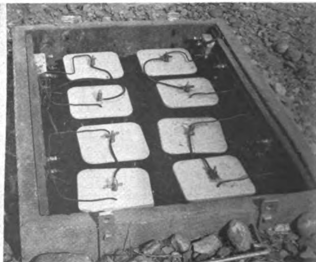
Storage battery supplies power for code units and switch machines; primary battery supplies track circuits
