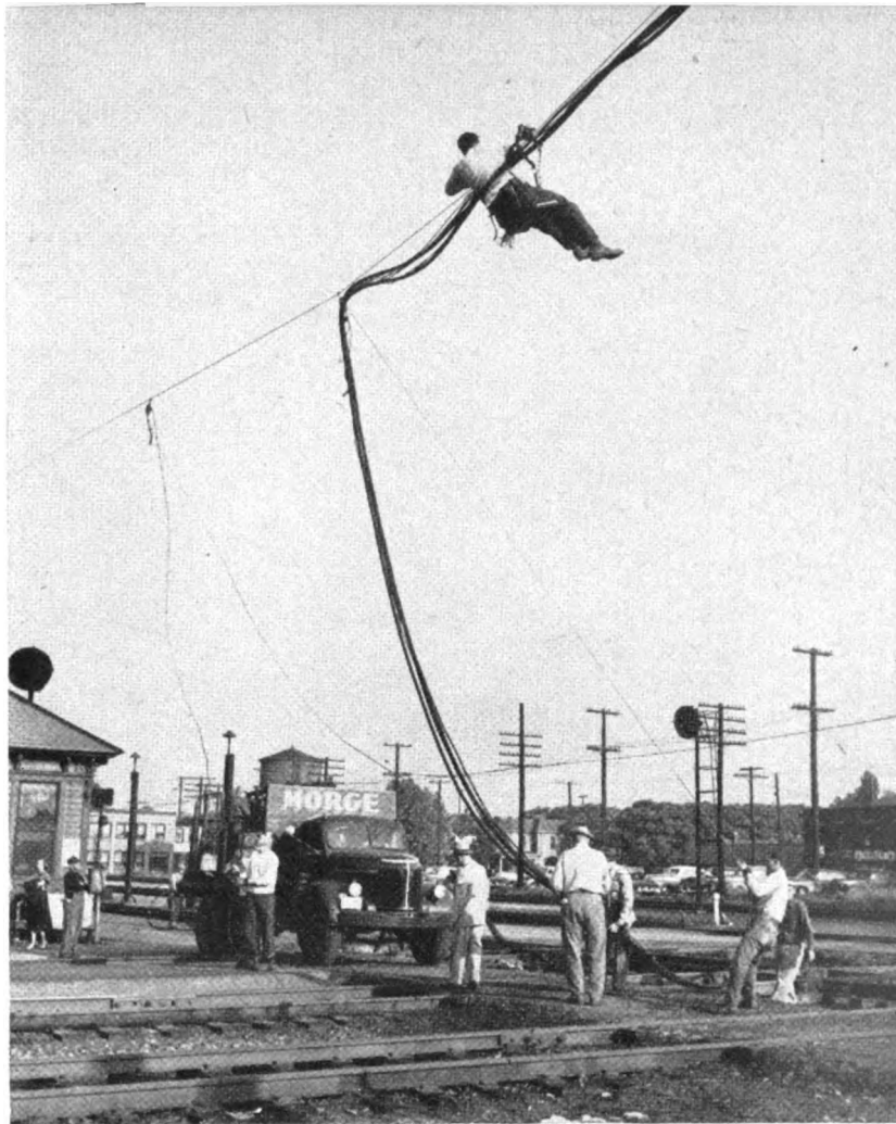
Throughout entire moving program the control machine was connected for normal operation by flexible cables
