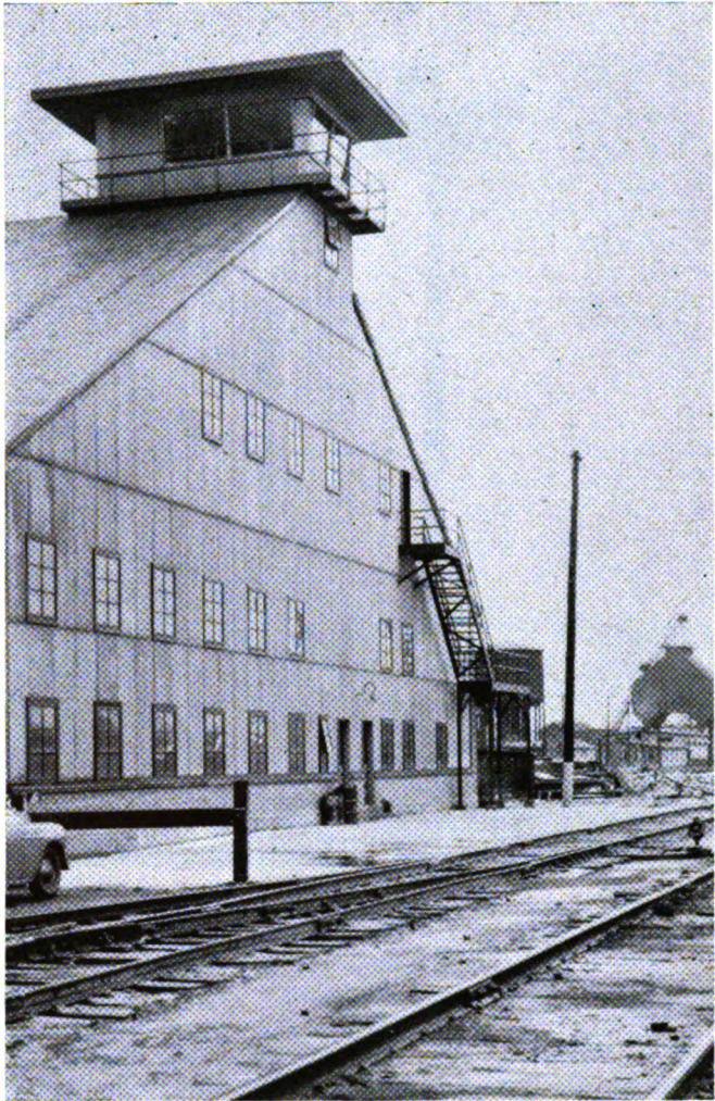
The yardmaster's office is on top of a tower 52 ft. above the ground
