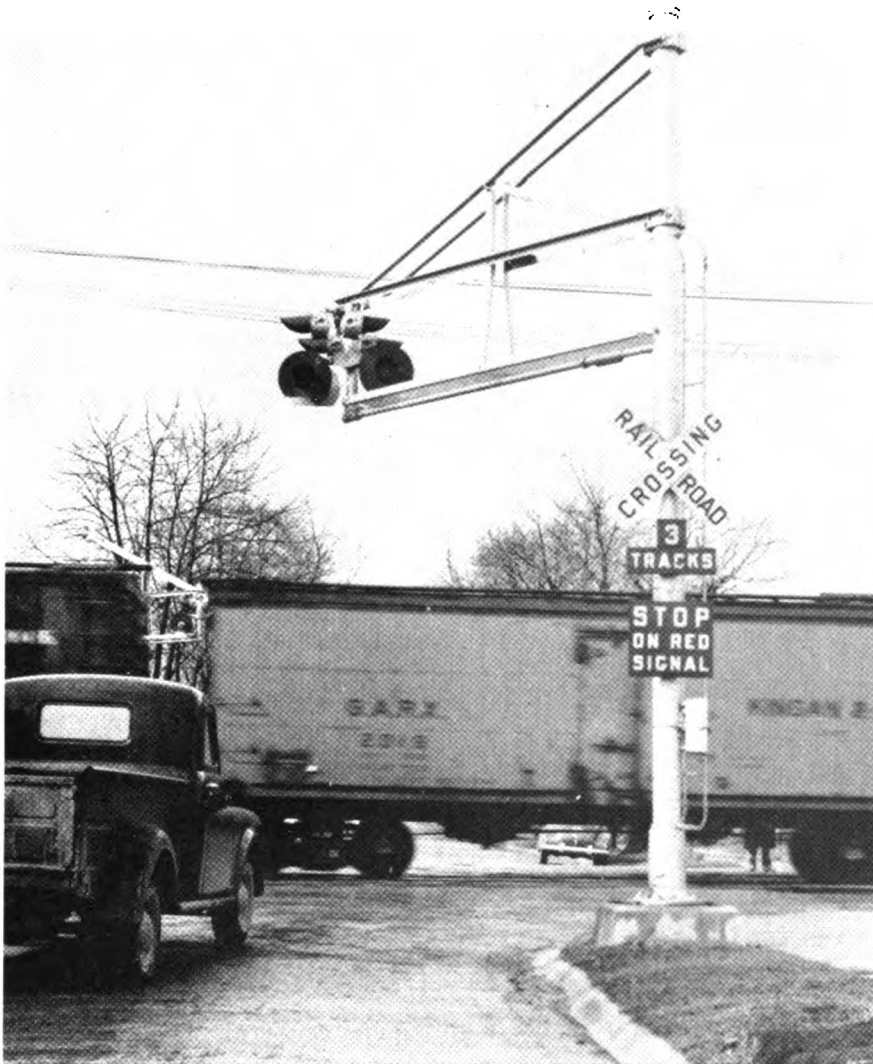
Cantilever extends out at 45 deg. over two streets which cross at 90 deg.
