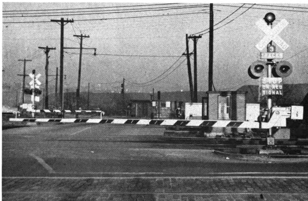
Gates lowered at the River Street crossing. Watchman's shelter is immediately to the left of right-hand gate and flasher
