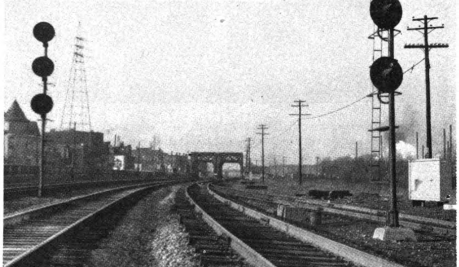
Above—The new signals are the searchlight type. Westward signal L108 is at right
