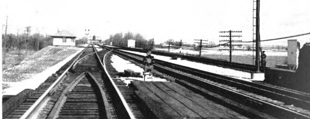
Interlocking at North Dayton, Ohio, with new bridge and track changes, replaces two hand-throw switch layouts
