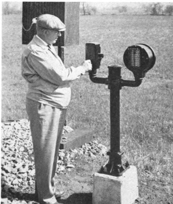
At a hand-thrown switch a conductor observes indicator and then uses key in controller to start time release
