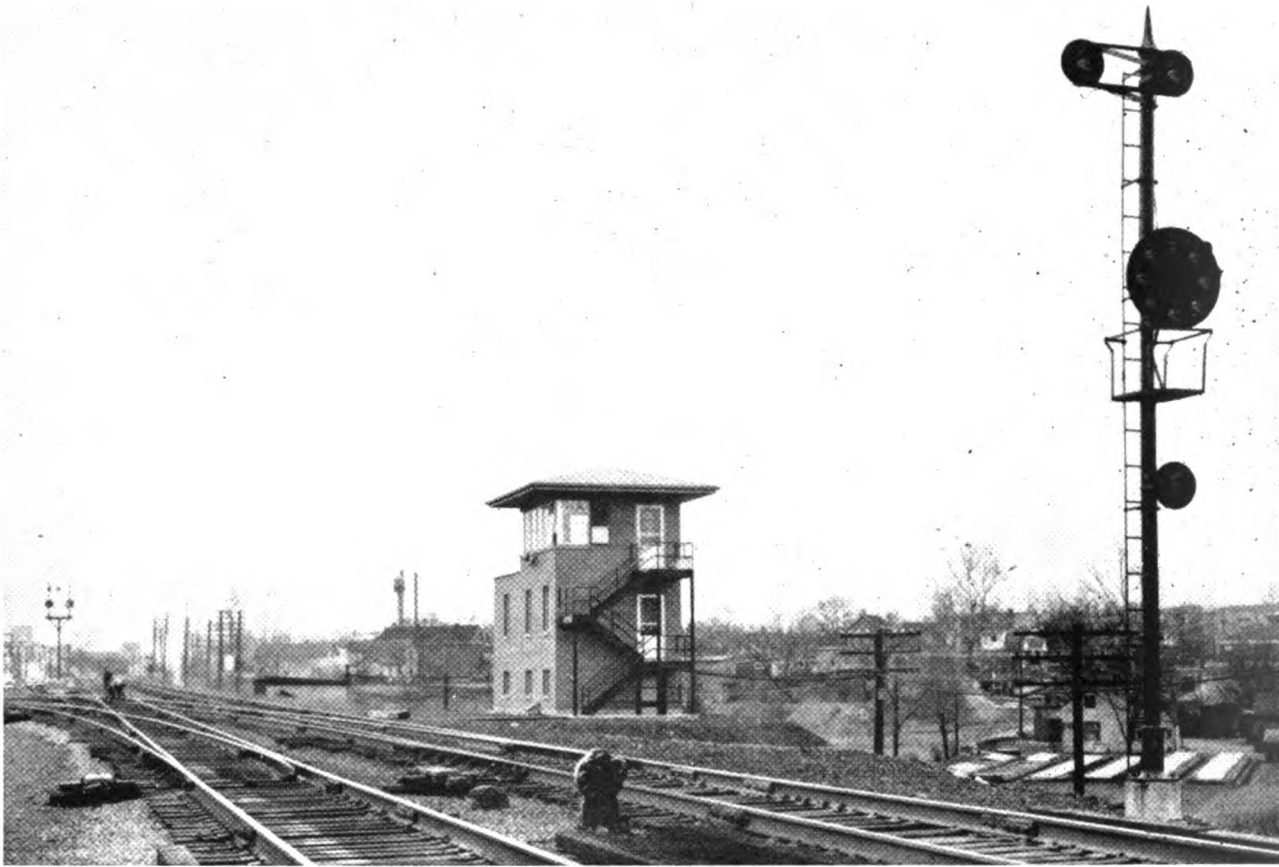
General view of the interlocking showing tower and eastward signals
