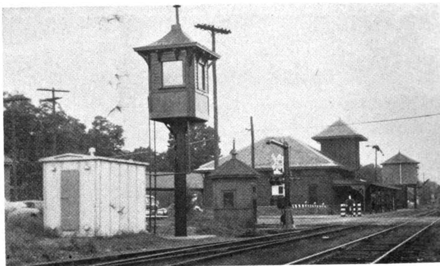
View of concrete house and control tower at Central Avenue
