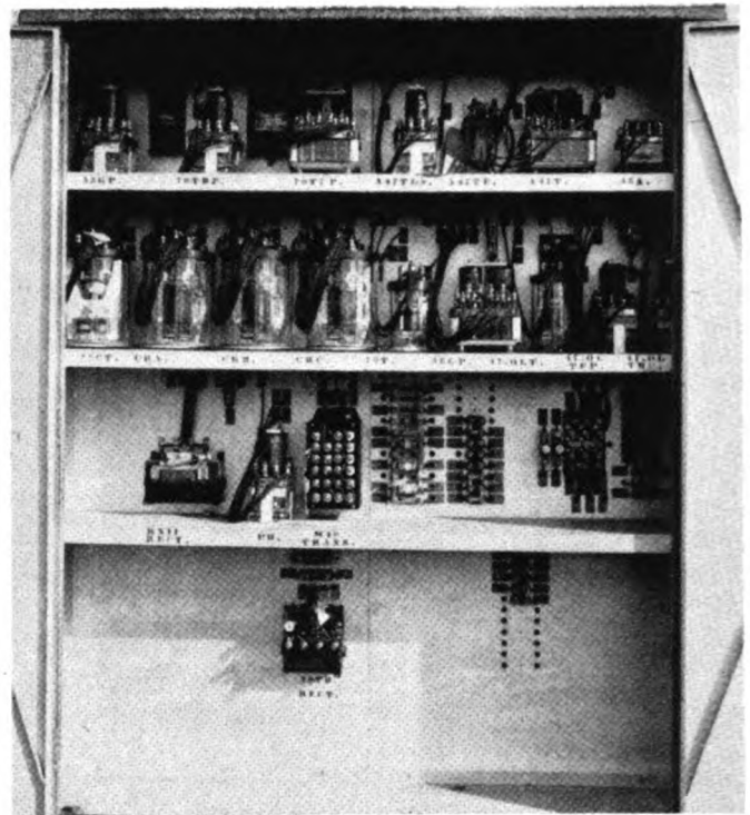
The relays including those for the coded track circuits are in cases
