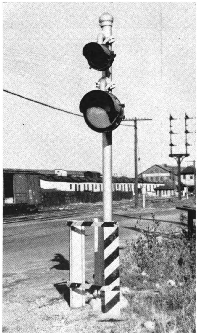
"No-Left-Turn" sign and yellow flasher in industrial driveway into First Street. Note scrap steel rail barricade painted black and white around base of mast
