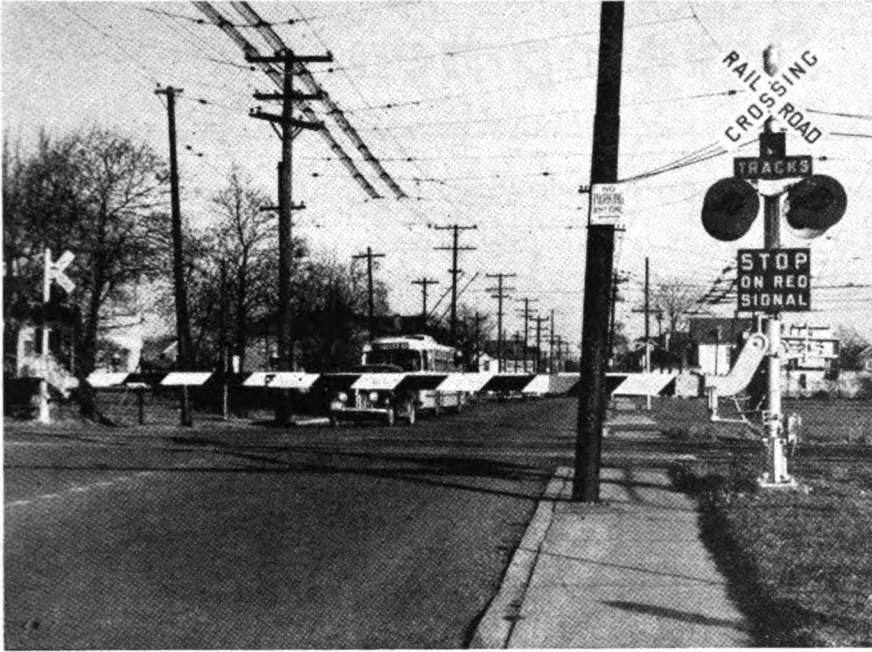
Gates and flashers at Bolander Avenue, showing gates lowered
