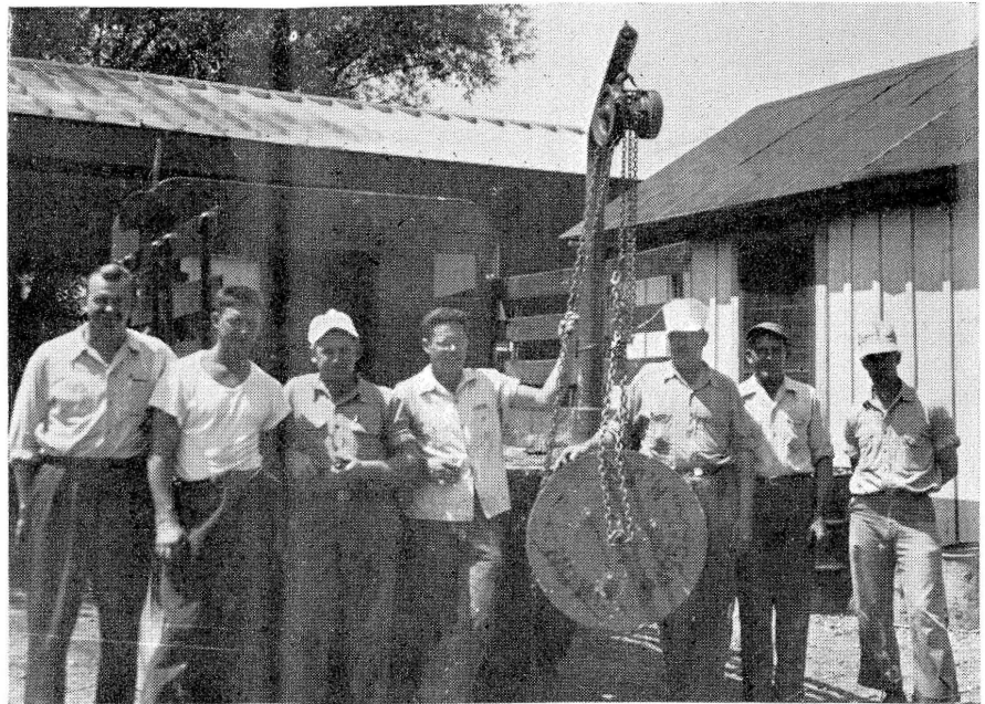
This crew installed the new street crossing protection
