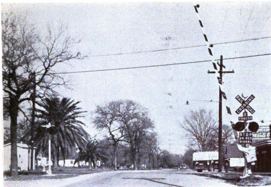
View looking north on northward driveway of the Heights boulevard showing gate at right and second flashing-light signal at the left of this pavement
