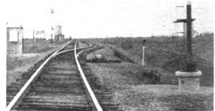
Station-entering signal at Corbin
