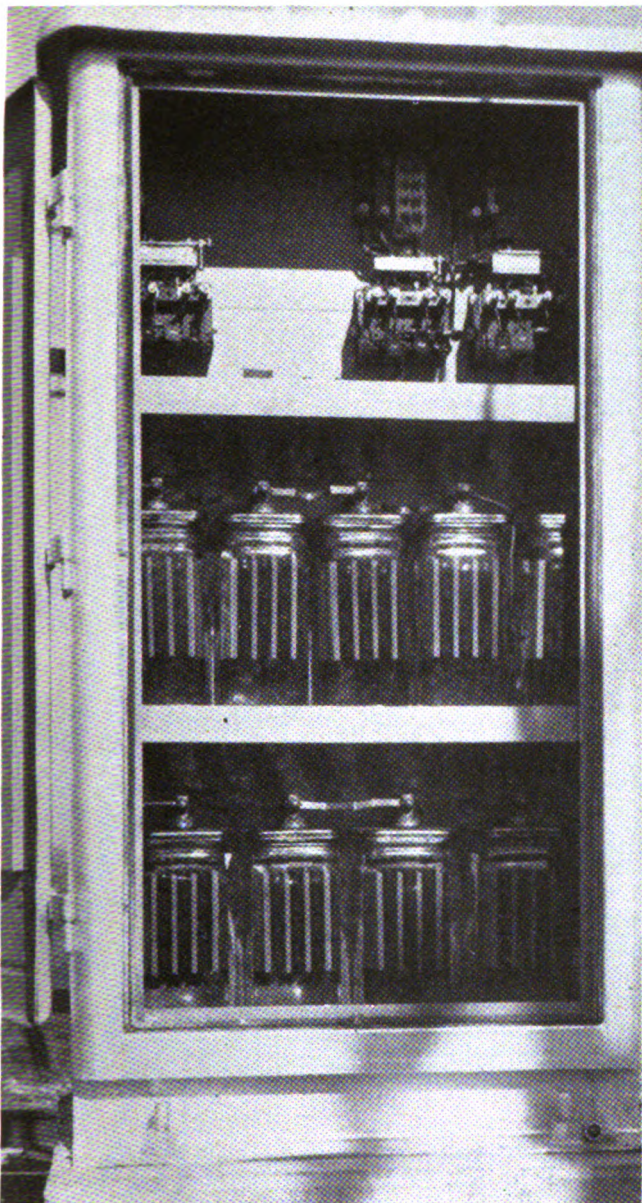
Left—Field side of a typical case at signal, showing storage batteries and the rectifiers
