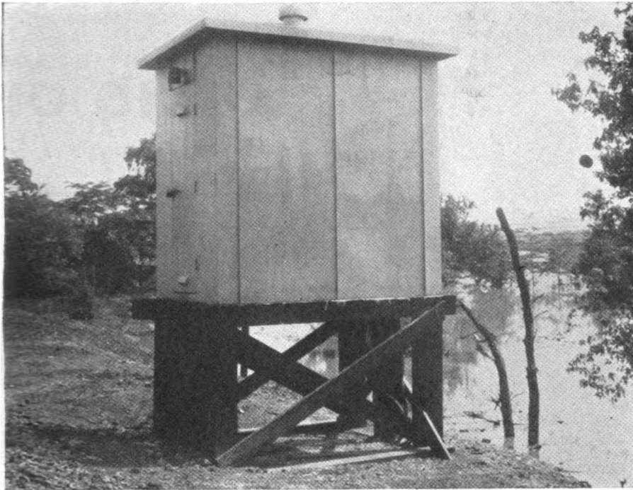
Bungalow on high timbers at the north end of King for flood protection
