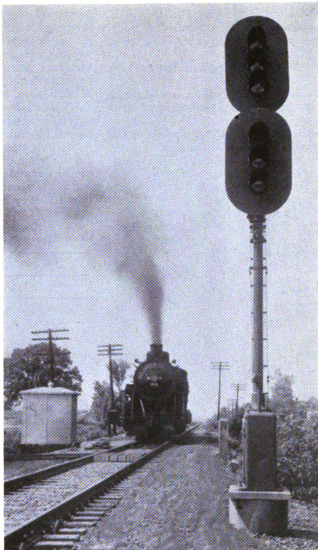
Typical C.T.C. controlled station-entering signal with two color-light type heads
