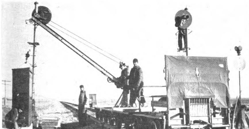
Rock Island uses crane on car to erect signals
