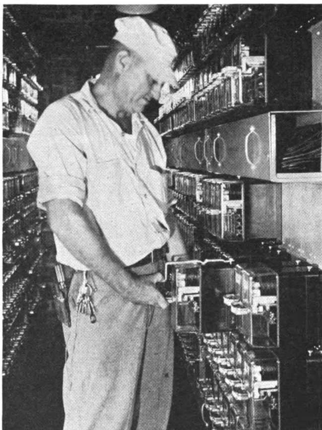
Signal maintainer replacing a plug-in relay
