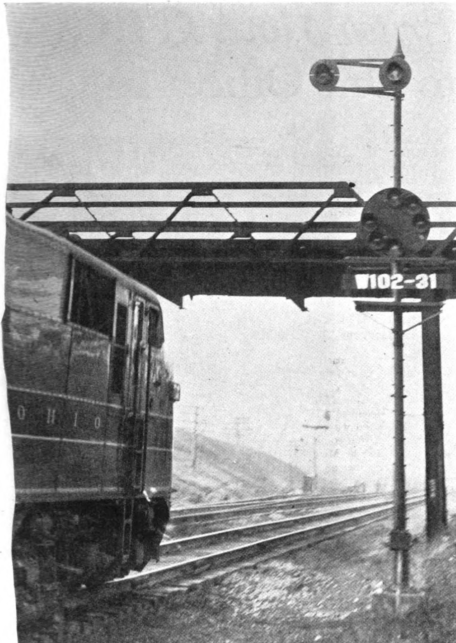
Westbound train passing westward distant signal W102-31
