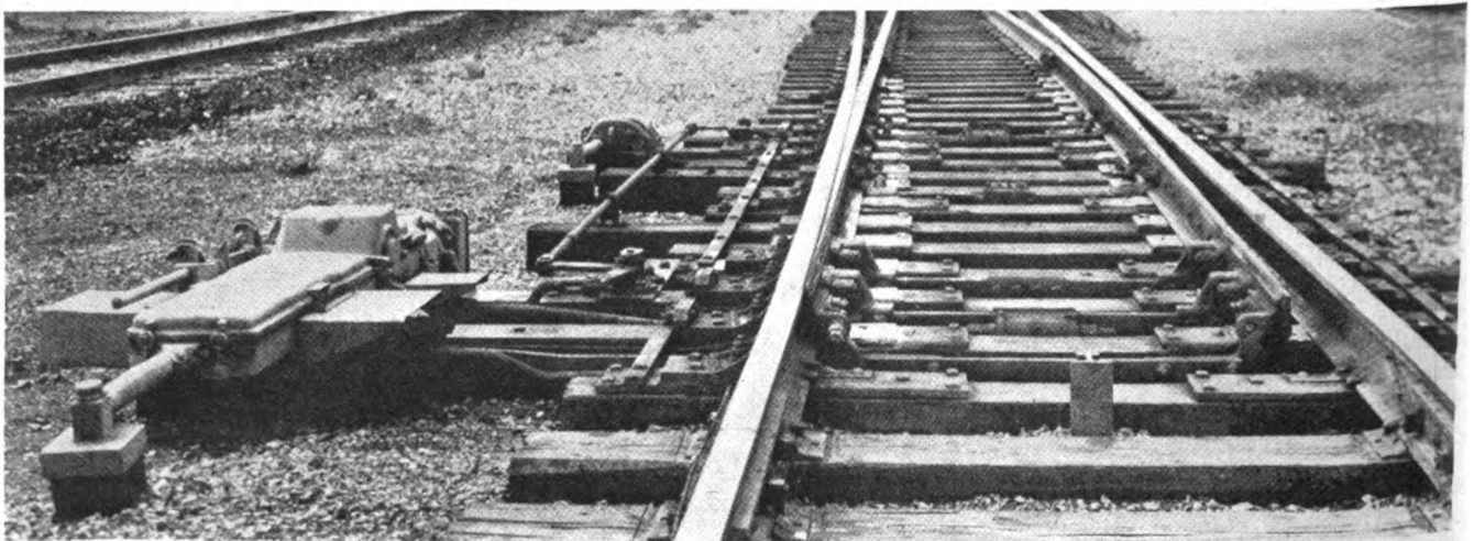
Power switch showing pipe and cranks for second connection to mid-section of the long points
