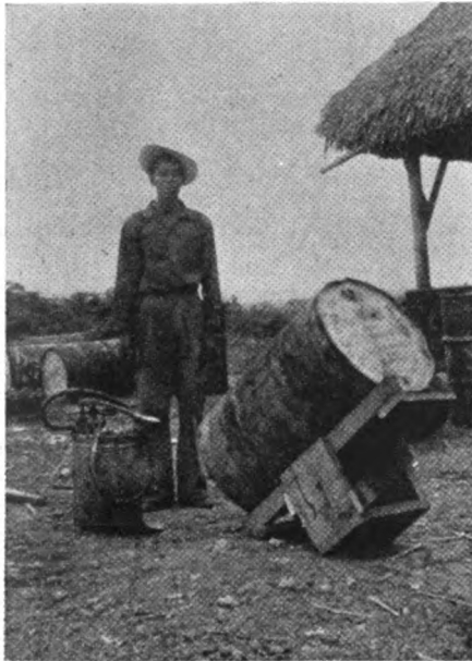
View showing a barrel in place on the cradle
