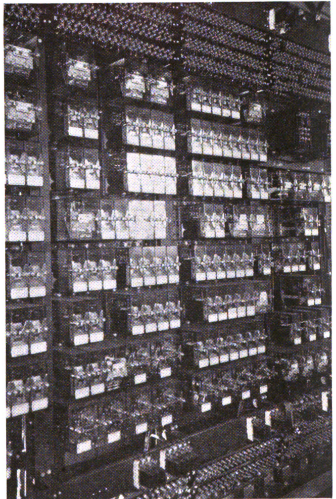
The relays in the house at Depew are the quick-detachable plug-in type
