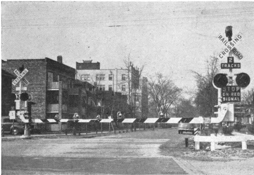
Typical short-arm gates and flashers on the Wabash in Gary
