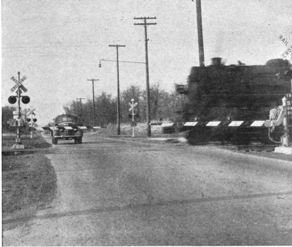
Typical installation of short-arm gates and flashers on the Michigan Central
