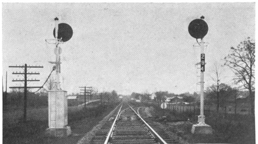
Typical station-entering signal at end of a passing track
