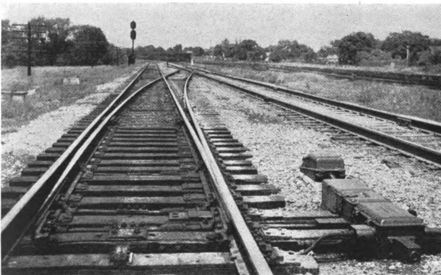
Crossover 17 on the C. & E.I. at North yard. Signal 18RA-B is in the background
