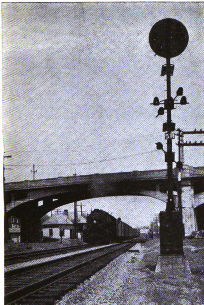
The signals on the Norfolk and Western are the position-light type. View shows high signal 5R
