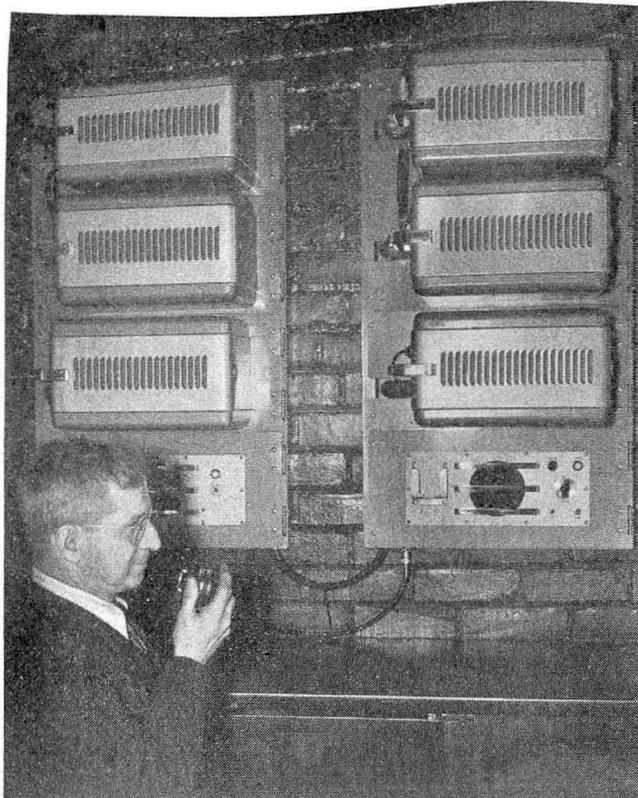
The satellite equipment at Dearborn. While this station operates unattended, it may be used as an originating station if desired.
