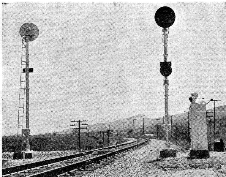
Intermediate signal with lower normally-extinguished green lamp unit. Right—Eastbound train at the east end of the Redlands siding
