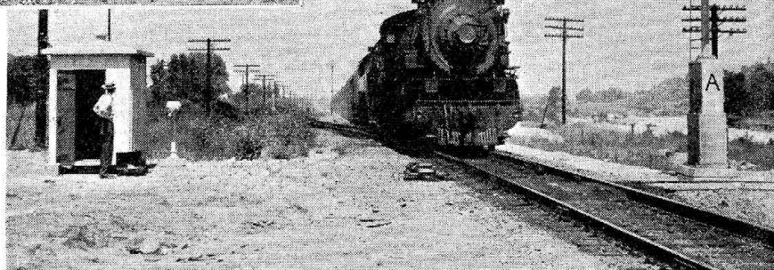
Intermediate signal with lower normally-extinguished green lamp unit. Right—Eastbound train at the east end of the Redlands siding
