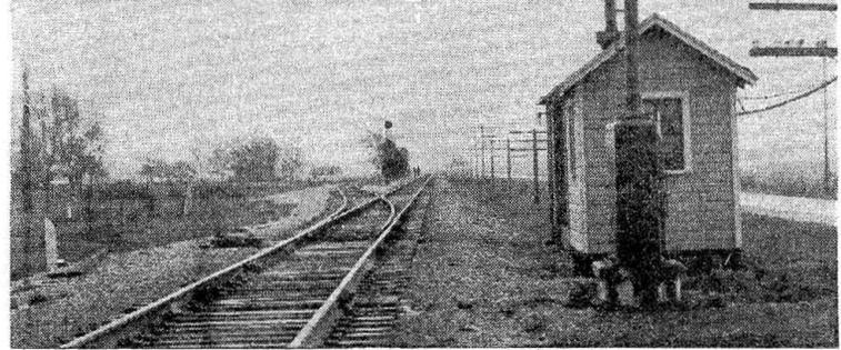
Above—Typical layout at end of power siding, the new frame building is for shelter of trackman when on duty to clean snow from the power switch
