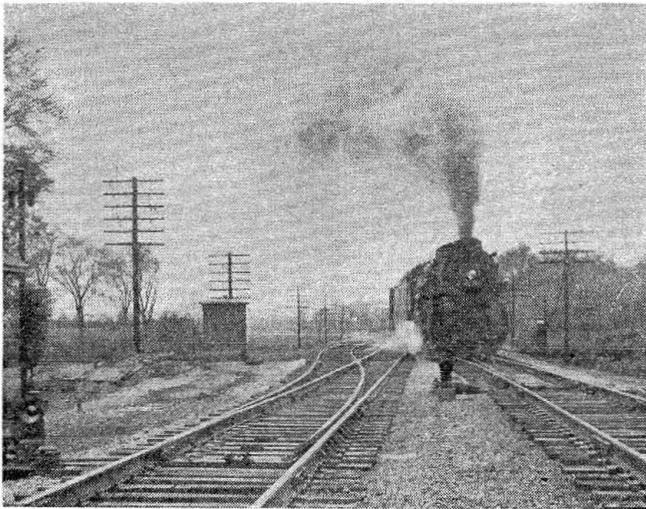
View looking west with an eastbound train using crossover 20, hand-throw yard switch at the left with two lamps on the post
