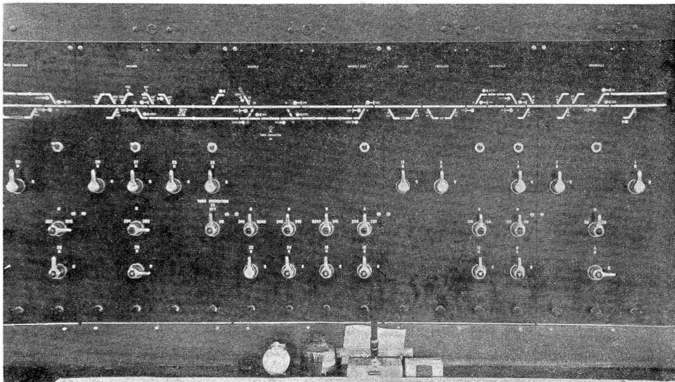
The C.T.C. control machine is located in the dispatcher's office at Waverly
