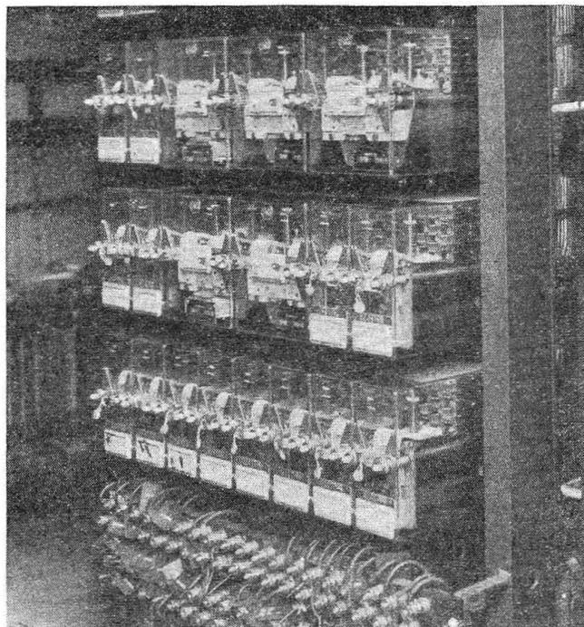
Quick-detachable plug-in relays mounted in rack in metal house
