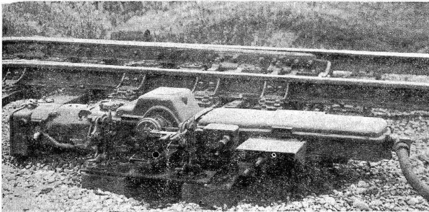
The electric switch machines are equipped for dual-control
