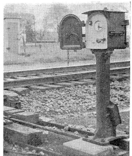
Electric lock on hand-throw switch in C.T.C. territory on the N.Y.C. & St. L.
