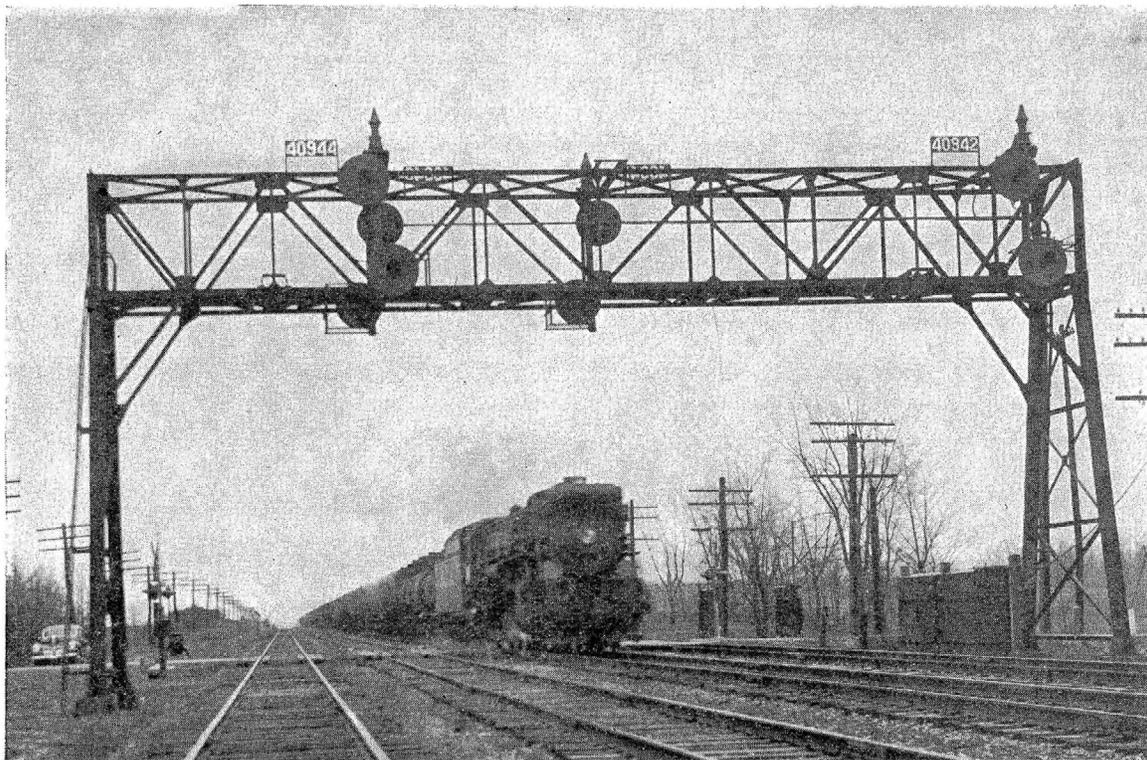
New search light signals with coded track circuits and no line circuits replace semaphores on the New York Central
