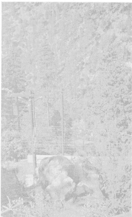
Pole line down mountainside
