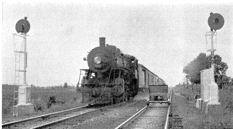
In 1942, the Louisville & Nashville installed double track automatic block signaling using coded track circuits and with no line wires
