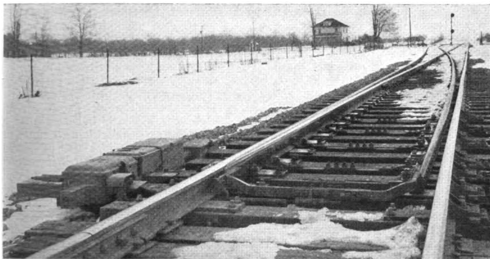
Left—Power switch at west end of Johnsons. Below—Semi-automatic signal 18L at Johnsons
