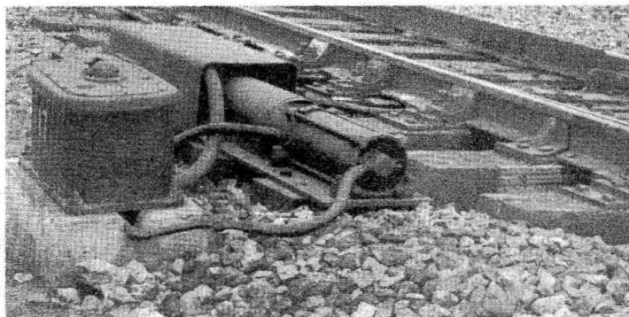
Above—Typical electro-pneumatic switch movement. Left—View looking north through subway with 16th street tower in foreground. Below—Signal 12R at 16th street plant
