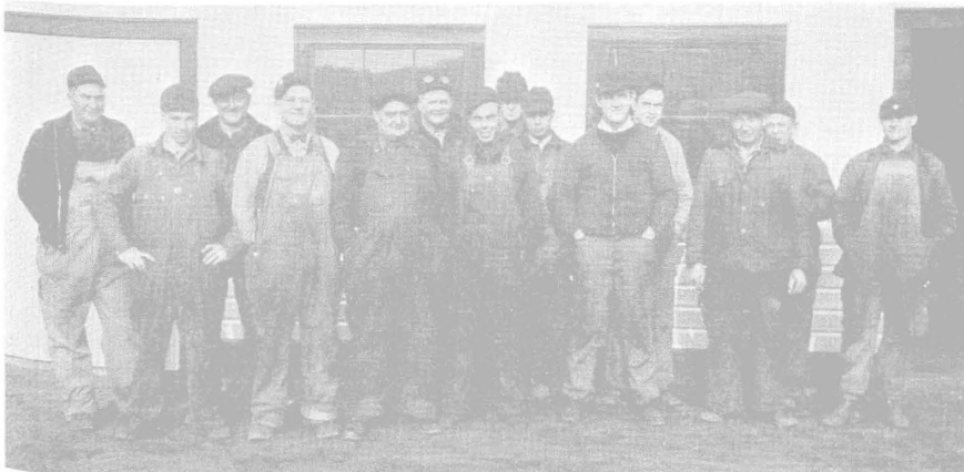
Signal construction gang at Clearing yard
