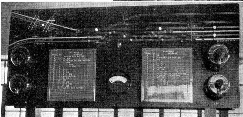
Above—Eastbound train passing westward home signal bridge. Left—Illuminated diagram, time-releases, and meter
