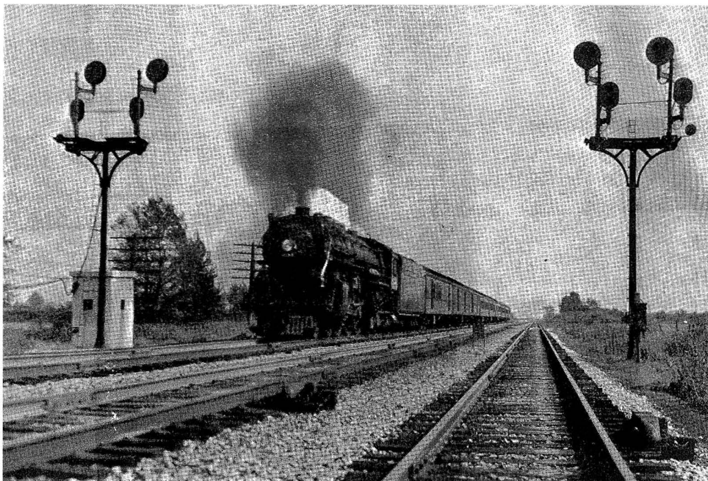
Typical signal location on four-track line showing the signals, inductors and the concrete house. Note the grade marker at the right
