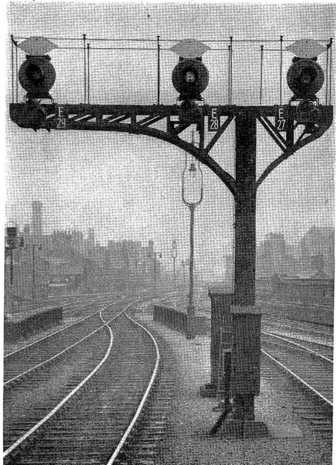
Bracket with three-aspect searchlight signals, and subsidiary signals
