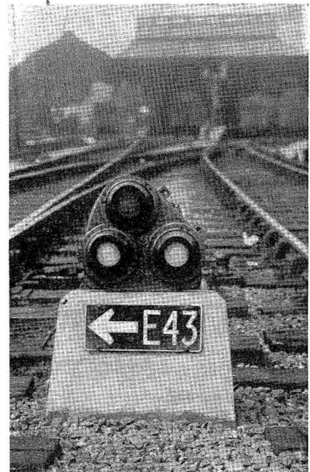
Position-light shunt signal
