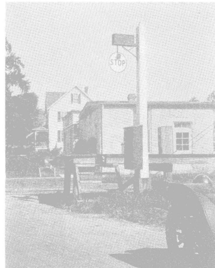
Adler rotating-disk signal installed on the Maryland & Pennsylvania at Glenarm, Md. on Feb. 25, 1921
