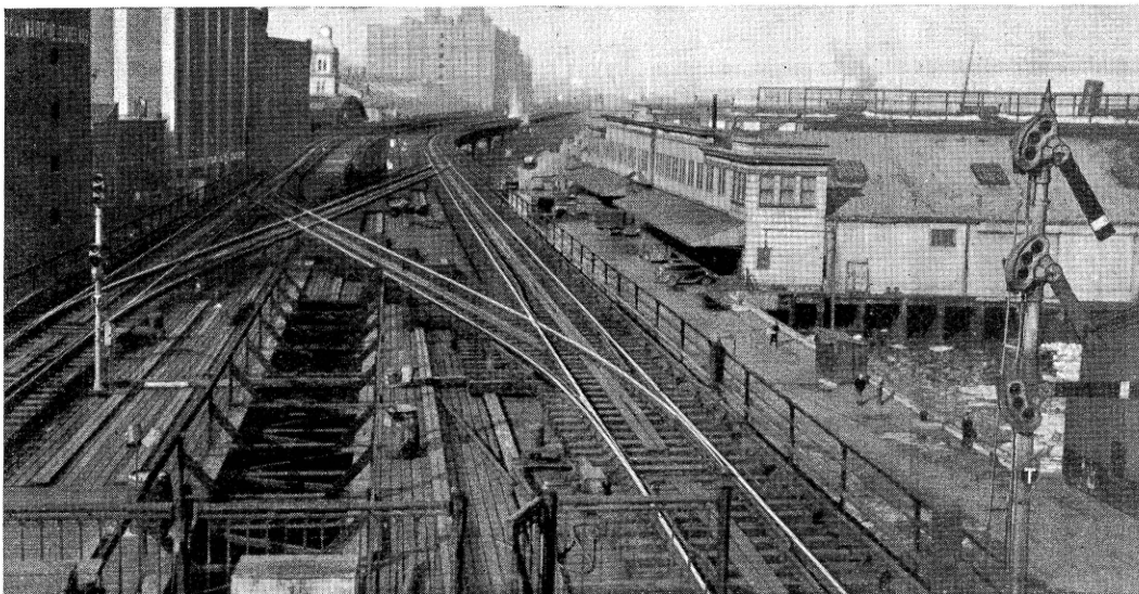
A mechanical plant involving switches for two crossovers on the Philadelphia Rapid Transit was replaced by an automatic control interlocking
