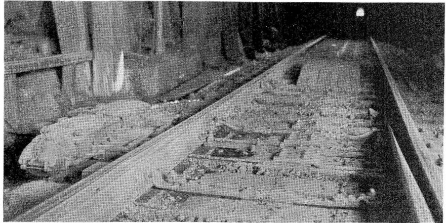
Switch layout and train-stop magnet in snow shed
