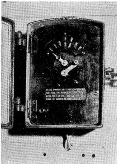
Alarm station with outer door open
