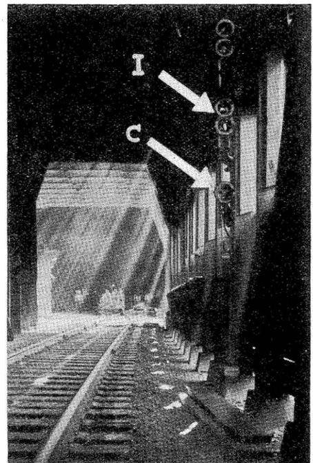
Call-on signal marked by arrow "C" and interlocking signal by "I"
