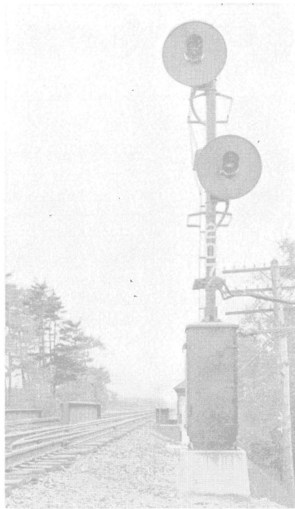
Two-unit multiple-aspect signal in approach to interlocking home signal
