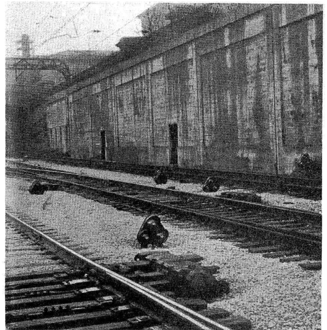
Color-light dwarf signals. Switch machines
