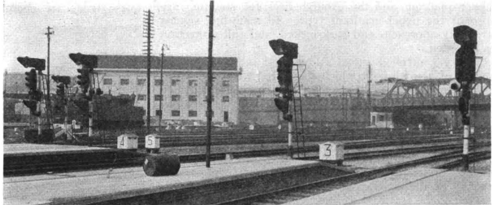
Three-aspect starting signals, with two-aspect shunt signals and optical route indicators
