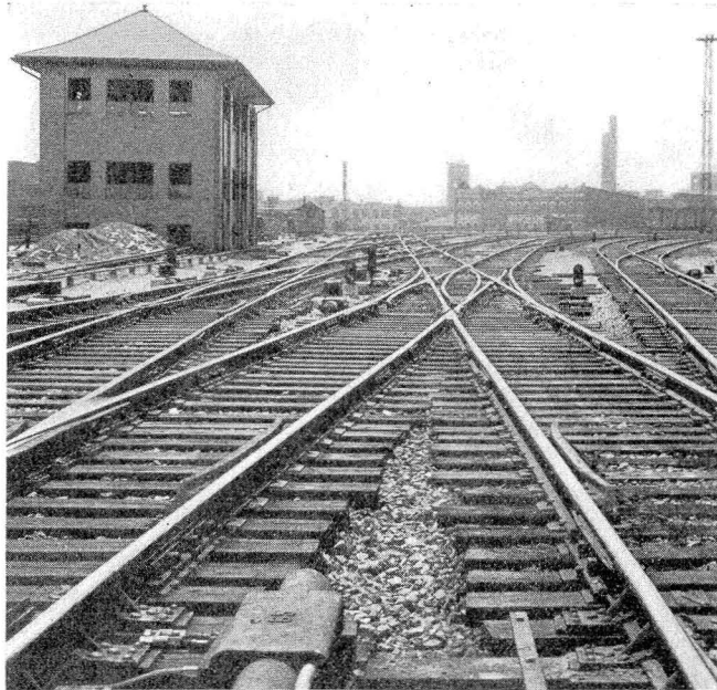
Tracks adjacent to the interlocking tower
