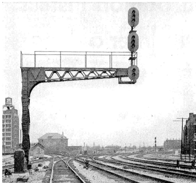
Color-light signals are used within interlocking limits
