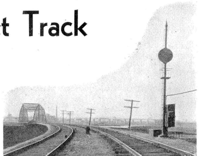
The dwarf signals are fixed in the stop position
