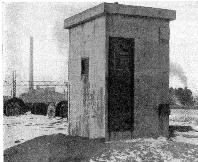
Type of concrete relay shelter which N. Y. C. is now using
