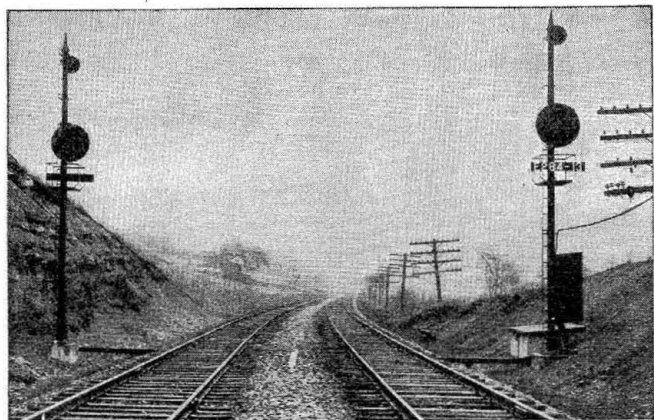
Signaling on the double track west of Grafton
