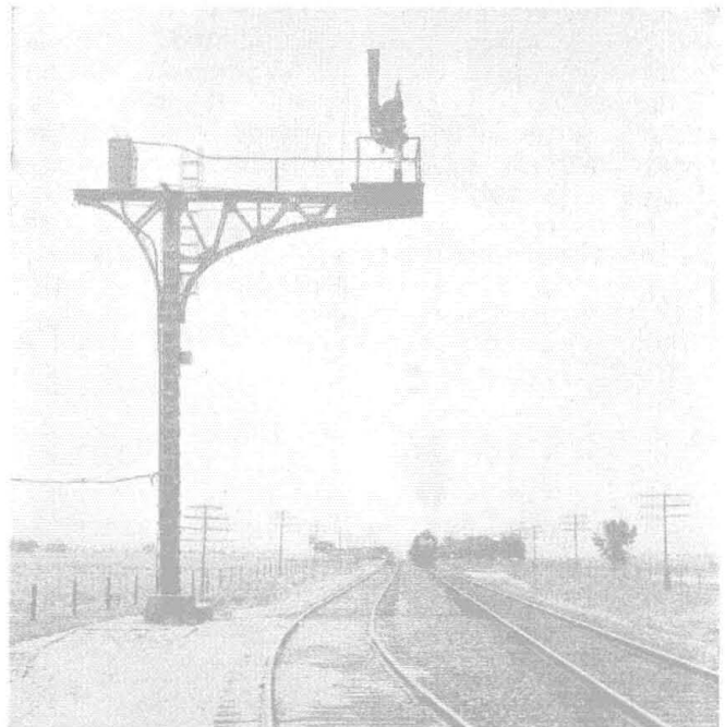
Recent semaphore signaling on the Coast Lines of the Atchison, Topeka & Santa Fe
